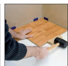
adjusting tongue-and-groove wood flooring boards.
